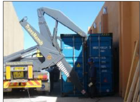
Container is set
