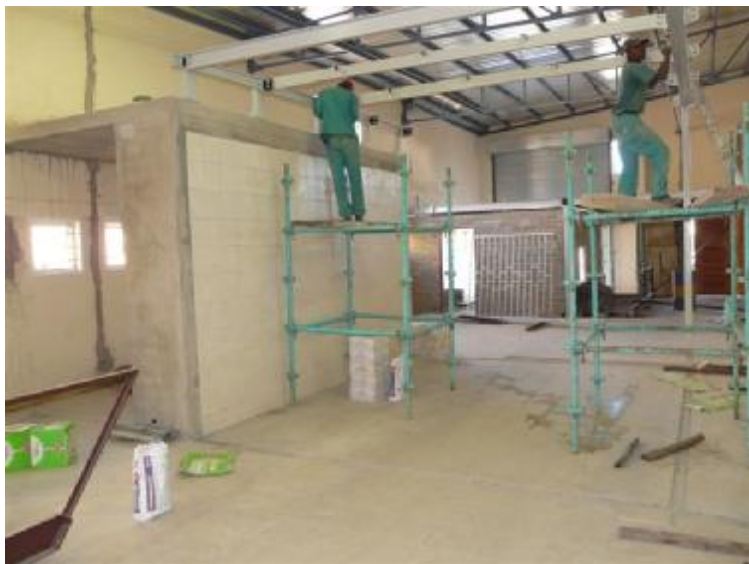
Steel construction Mezzanine Floor (above) and fermenting room (left)
