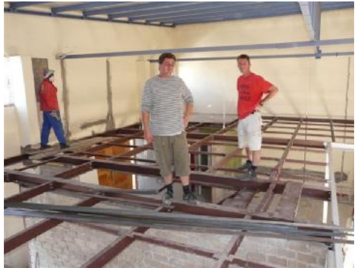
Steel construction Mezzanine Floor (above) and fermenting room (left)
