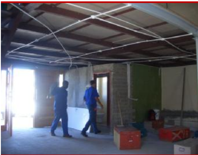
Steel construction Mezzanine Floor in April and early May 2009
